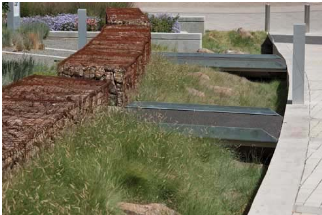
Here's a closer look at the metal deck bridges across the planted swales. Various seed mixes, blue grama prominent here, were developed and used to restore the disturbed shortgrass prairie landscape and unite the site with the area's mesa geography.
